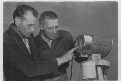
CHECKING ONE of the three air sampling filters atop Corporation buildings are Allen Hobbs, left, and Garvey Pierson, both of 3161, Industrial Hygiene Division. Sampling of air is part of the national "Fall-Out Network" in action during OPERATION TEAPOT at Nevada Test Site.
